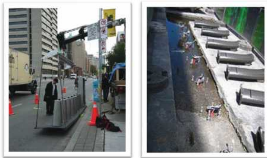
Figure 12: Modular stations placed at location pre-determined in New York & Excavation and trenching required for fixed stations (Source: “Bicycle Share opportunities in New York city”, NYPCPD)
